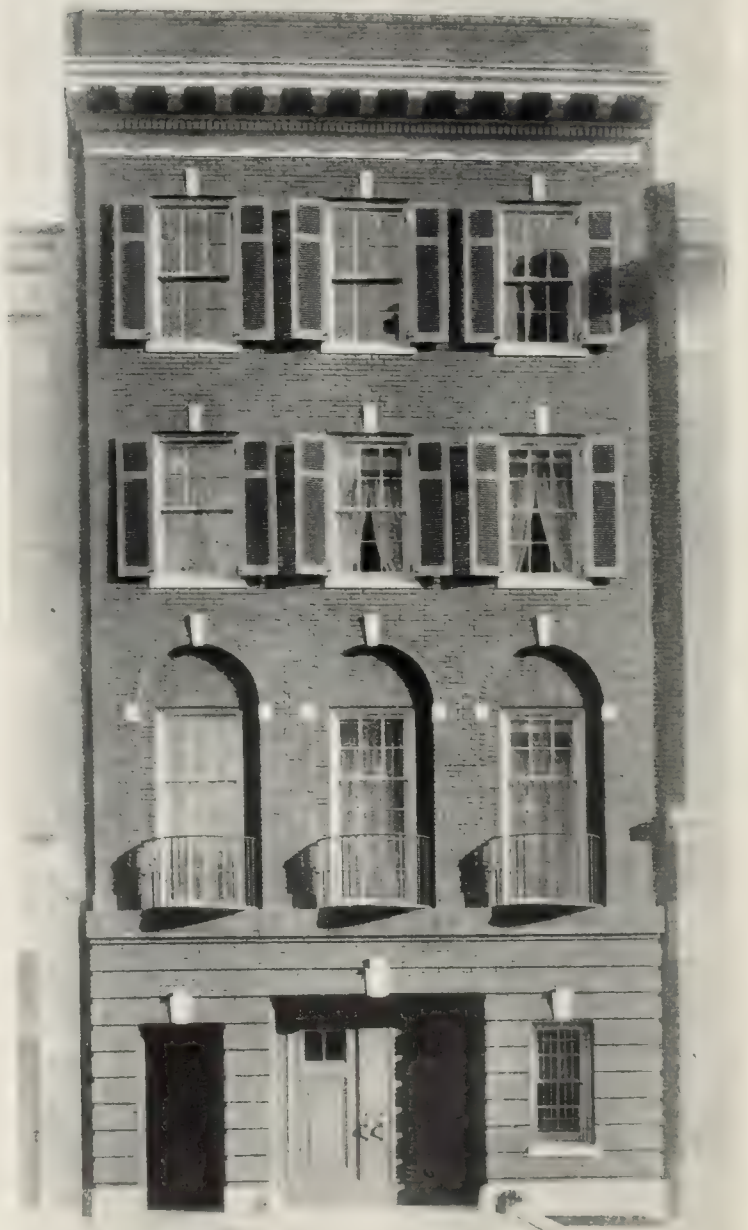
GARAGE AND APARTMENTS FOR RICHARD M. HOF, ESQ. 163 EAST 69TH STREET, NEW YORK CITY ALBRO & LINDBERG, ARCHITECTS
